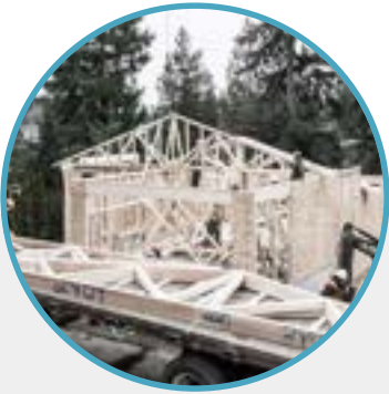
Single-Family Home Builders
